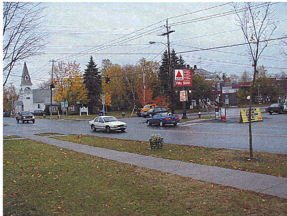
View to the Main Street/ Vermont RT 30 signalized intersection.
