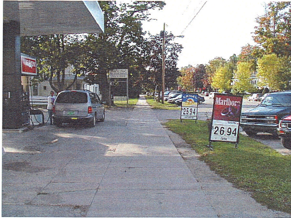
Exxon frontage on Main Street exemplifies recent automobile-oriented commercial development with driveways and parking in front. Circulating vehicles trying to get around the gas pumps are forced to illegally drive over the public sidewalks.
